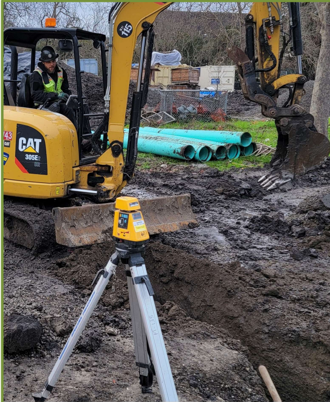
Storm Drain Trenching
