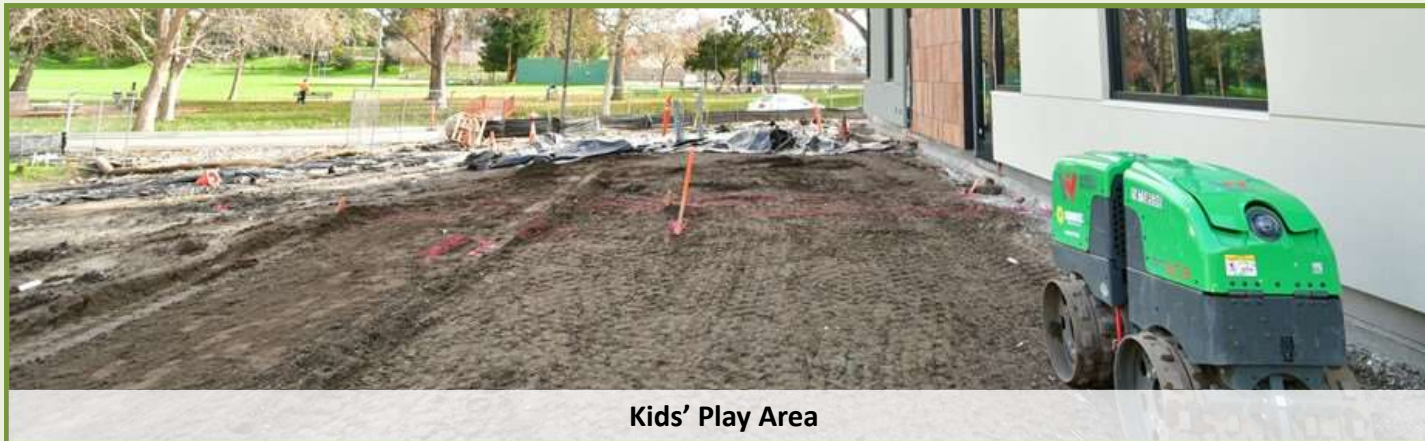
Kids' Play Area – Excavation of Fence Footing
