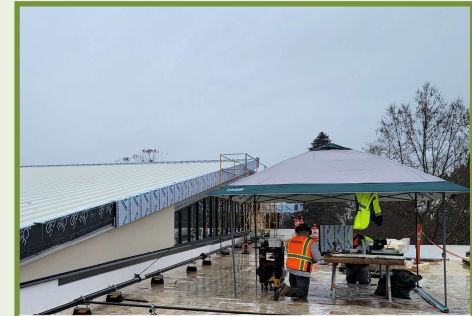
ACM Panel Installation
