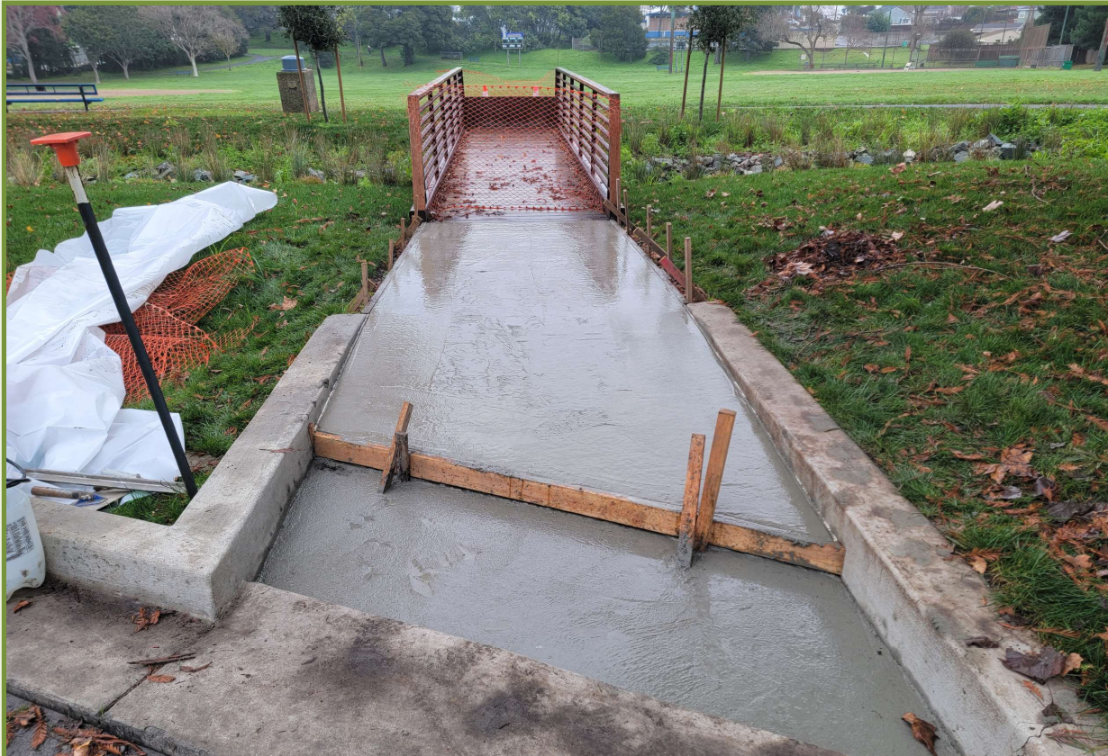
Pedestrian Bridge Approach
