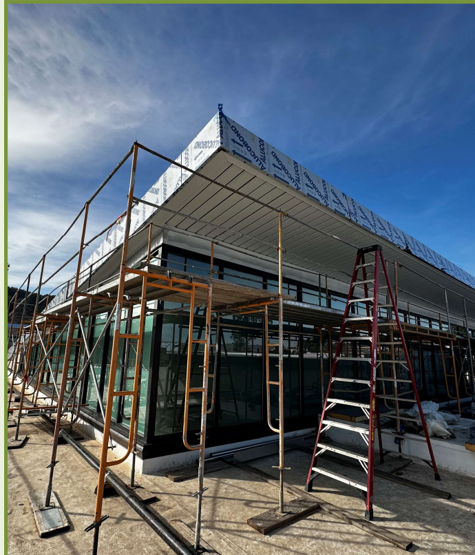
Gymnasium Clerestory Windows
