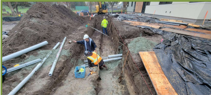
Kids' Play Area – Excavation of Fence Footing
