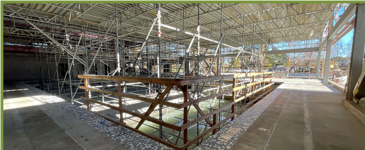
Indoor Pool Deck Poured
