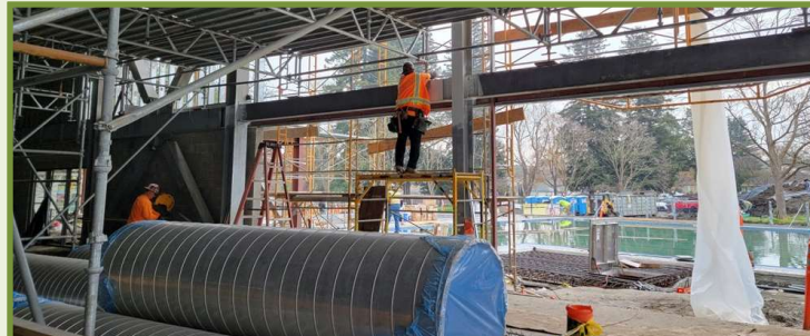
Framing of the Natatorium's West Wall
