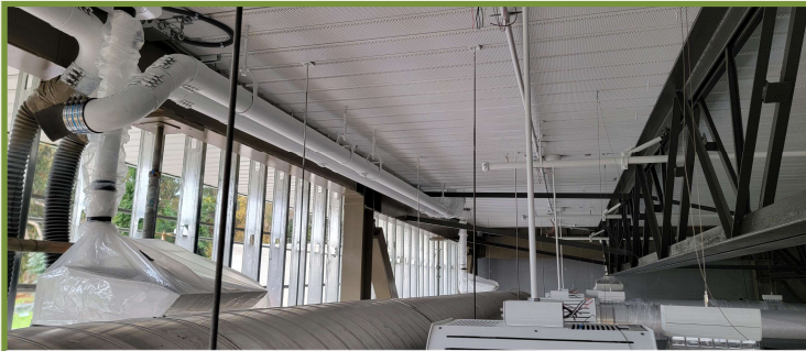
Natorium Ceiling Painting, MEPs, Lighting, and Fire Sprinklers
