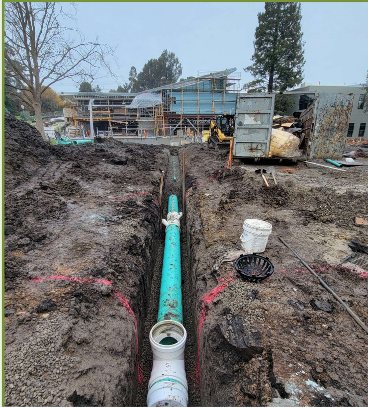
Storm Drain Trenching
