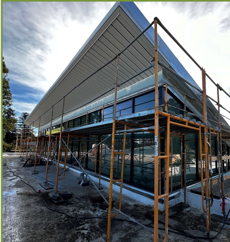
Natorium Clerestory Windows
