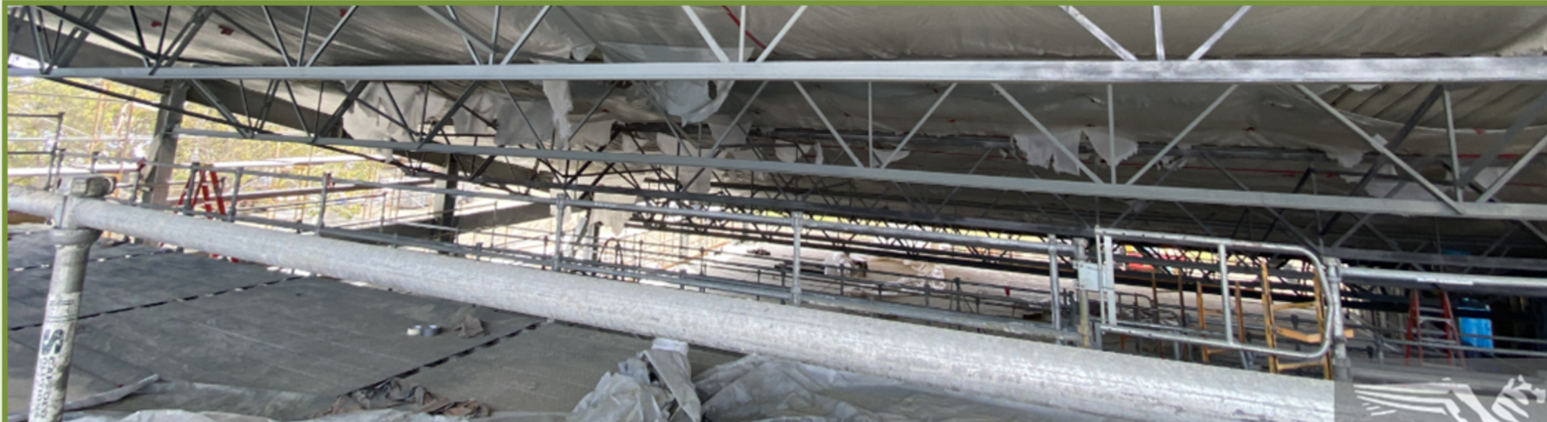
Natatorium Ceiling Work
