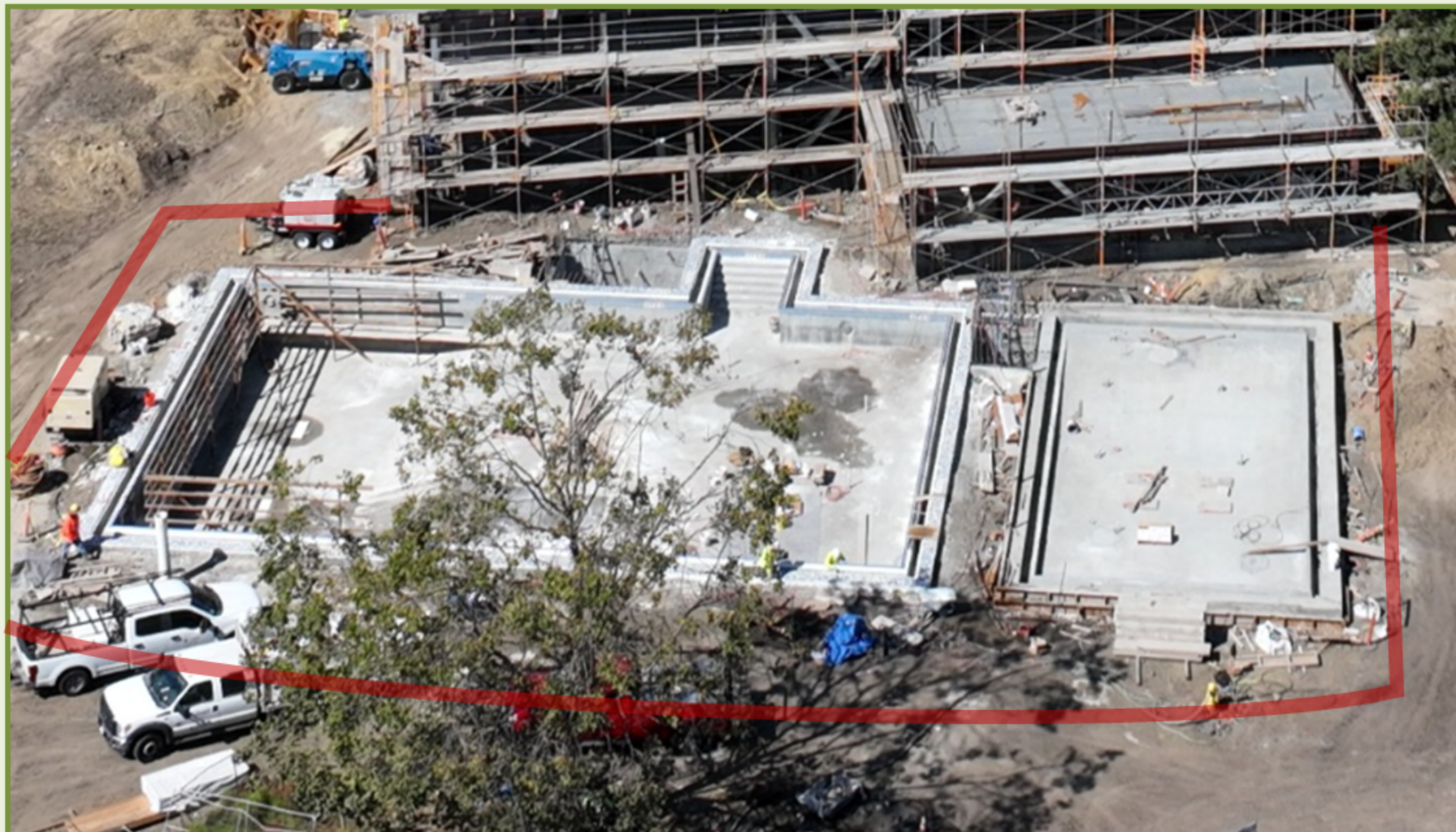
Retaining Wall and Outdoor Pools
