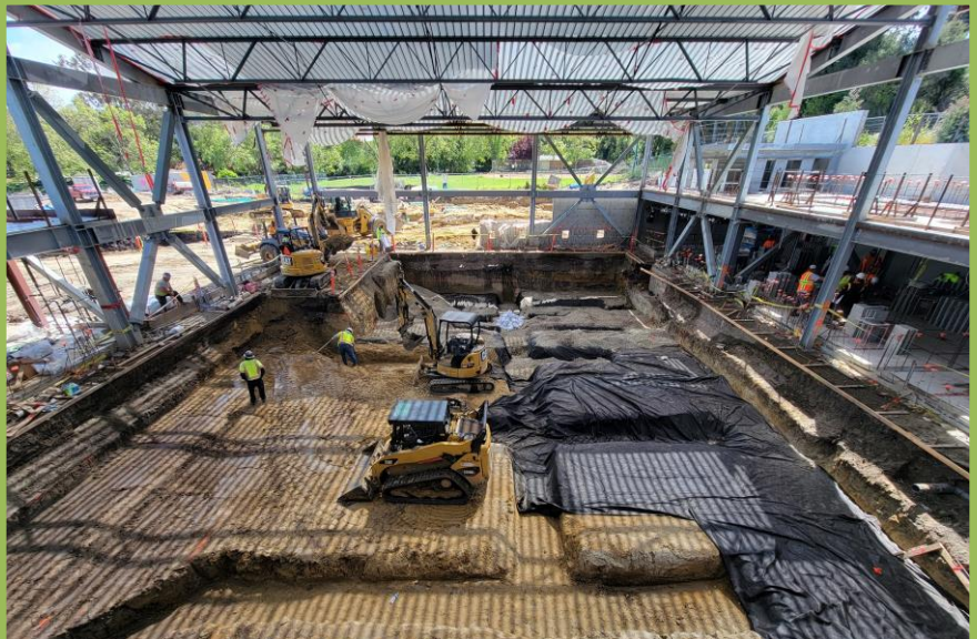
INDOOR POOL TRENCHES
