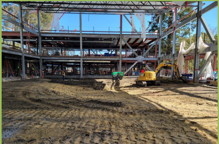
INDOOR POOL EXCAVATION
