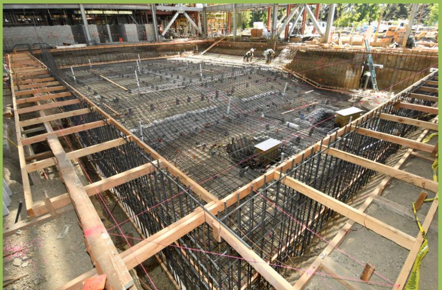
INDOOR POOL REBAR
