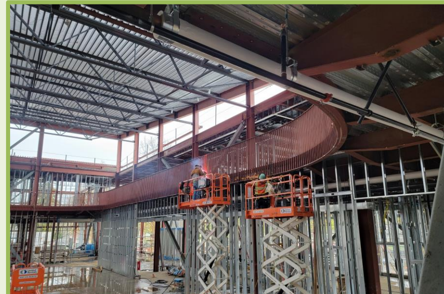
GUARDRAILS AT TRACK
