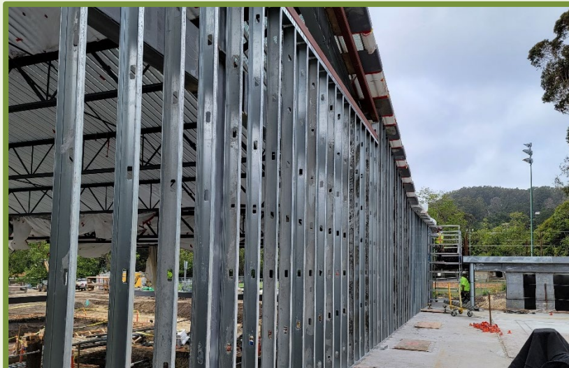
1 - EXTERIOR WALL FRAMING AT MECHANICAL ROOF
