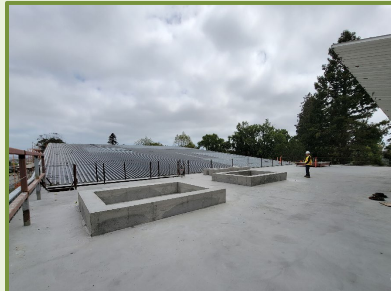
2 - Poured Flat Roof
