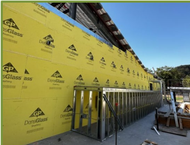
1 - EXTERIOR WALL SHEATHING AT MECHANICAL ROOF
