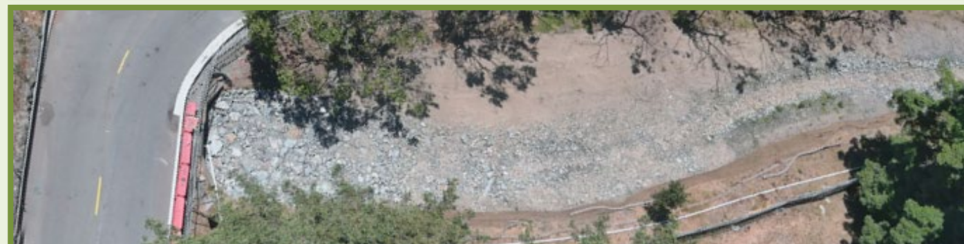
COMPLETED REPAIR AND MODIFICATION
