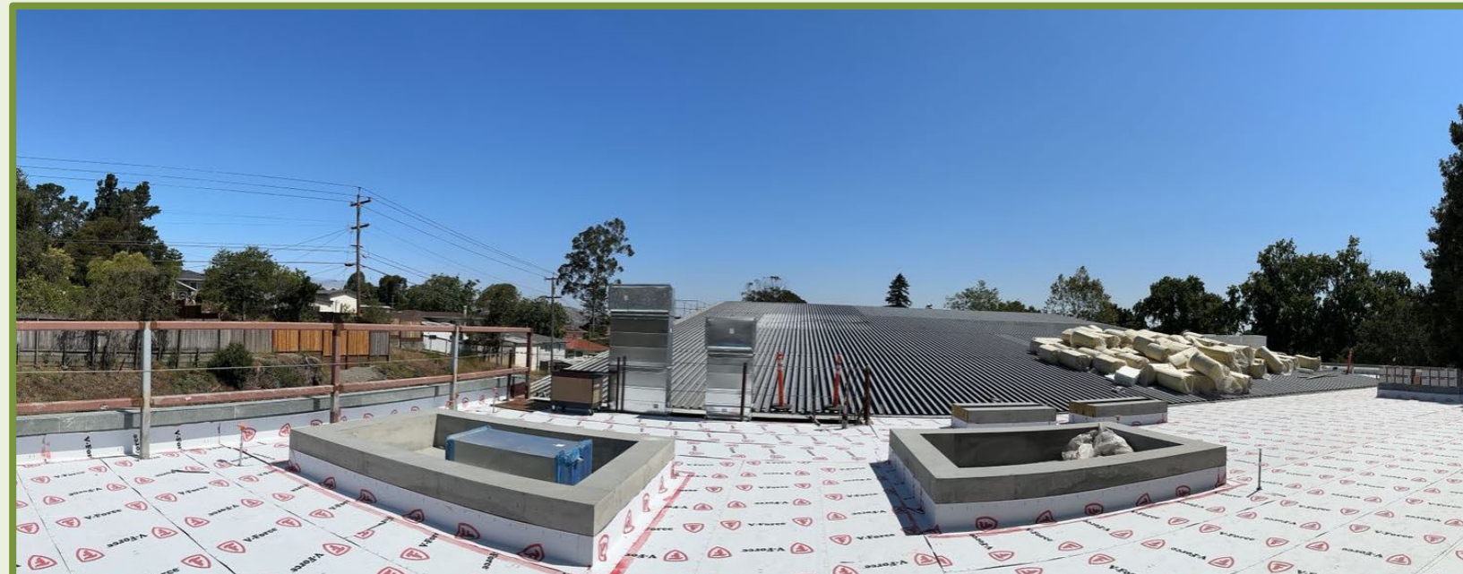
2 - VAPOR BARRIER INSTALLATION – FLAT ROOF
