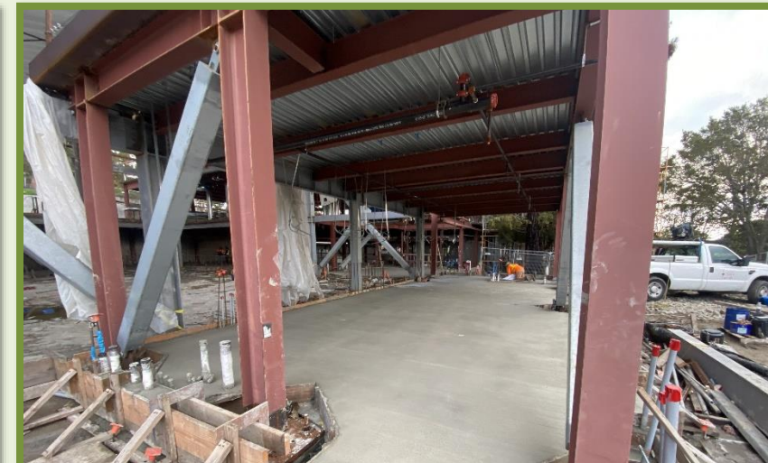
POURED CONCRETE SLAB (Party Rooms 1 & 2)
