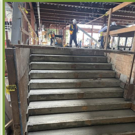
POURED STAIRS (To Locker Room From Gymnasium)
