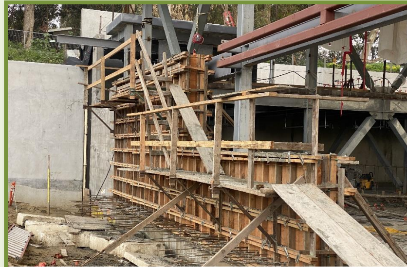
POURED LINE 1 CONCRETE WALL
