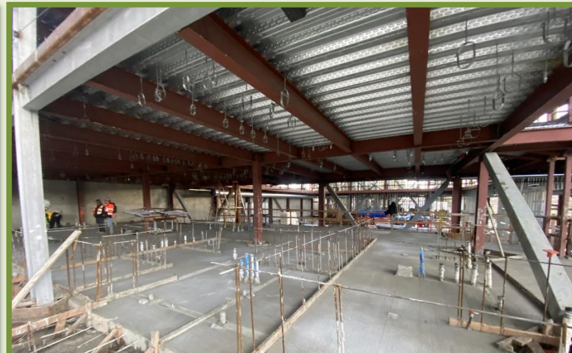
POURED CONCRETE SLAB (Women's Restroom, Men's Restroom & Showers)
