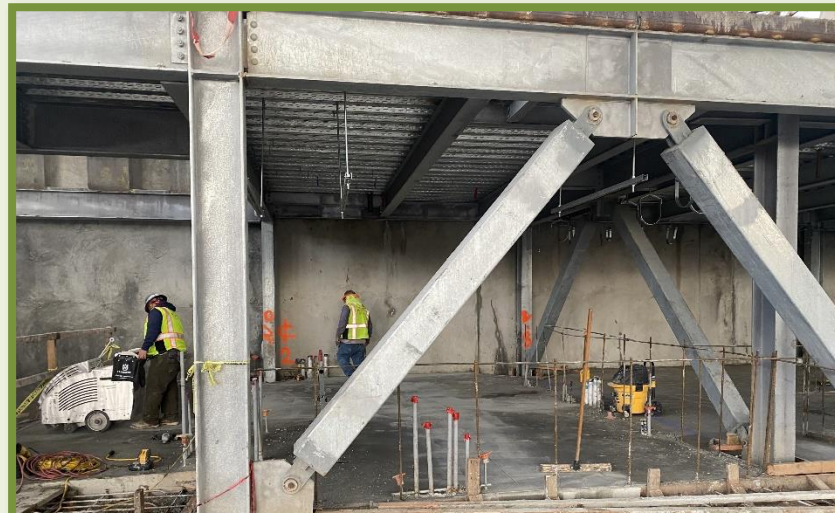
POURED CONCRETE SLAB (Pump Room & Pool Storage)
