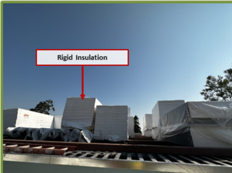
4 - Community Hall Roof Preparation
