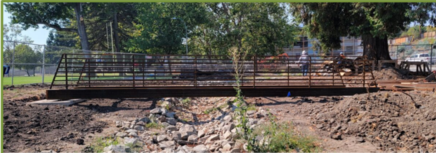
Mounted Pedestrian Bridge
