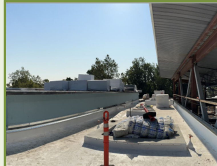
3 – Completed TPO Flat Roof
