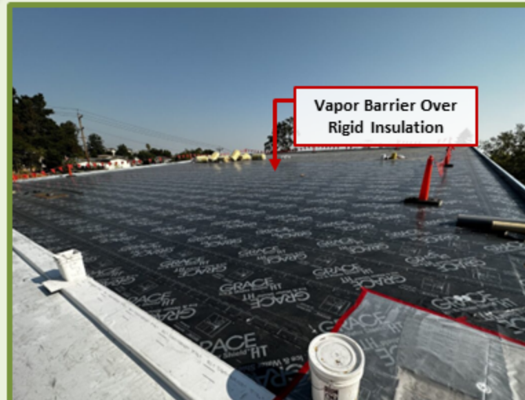
5 - Gymnasium High Roof
