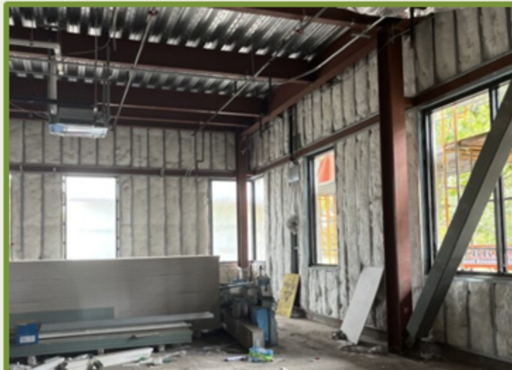
1 – Insulation and Window Work
