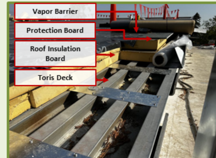
High Roof Cross Section
