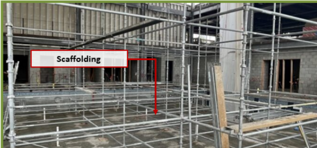
Scaffolding for Natatorium Ceiling/MEP
