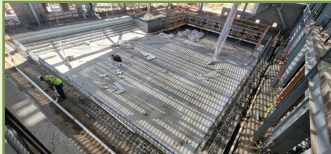
Completed Pool Shell - South
