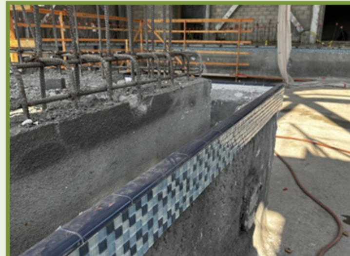
Tiling at Water Line
