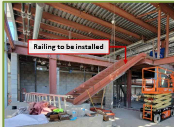
6 – Pool Lobby Stairs
