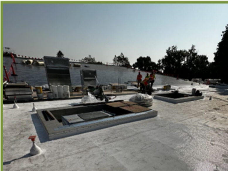
1 – Completed TPO Flat Roof
