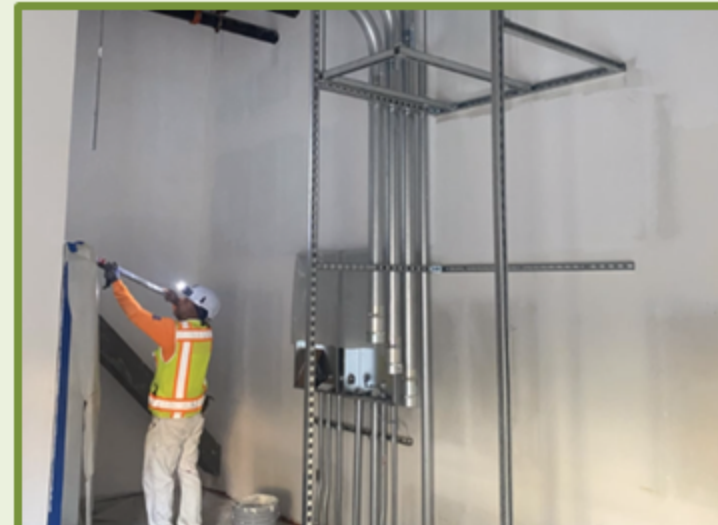
3 – Electrical Room Painting
