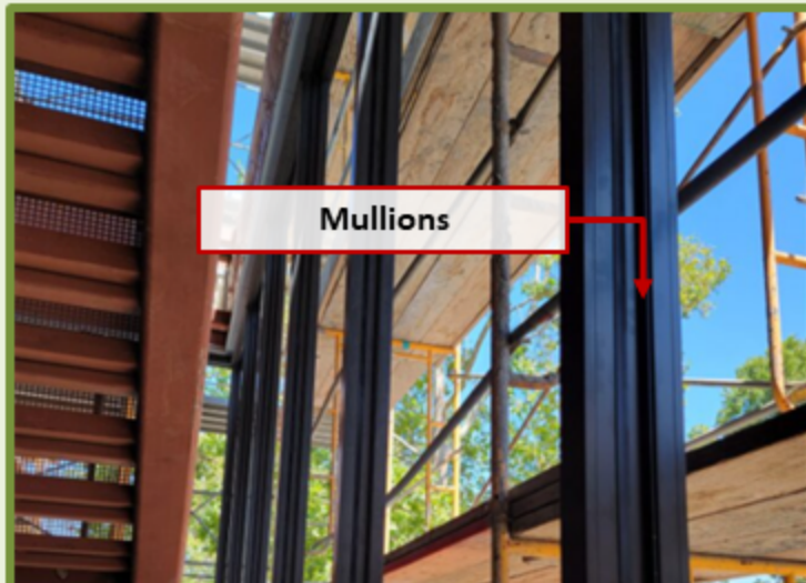
4 – Preparation for Windows
