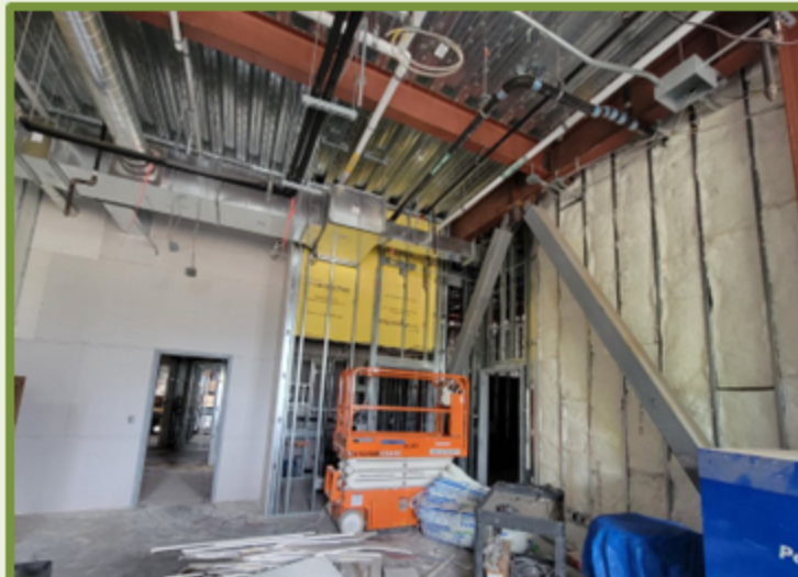
1 - Insulation - Small Classroom
