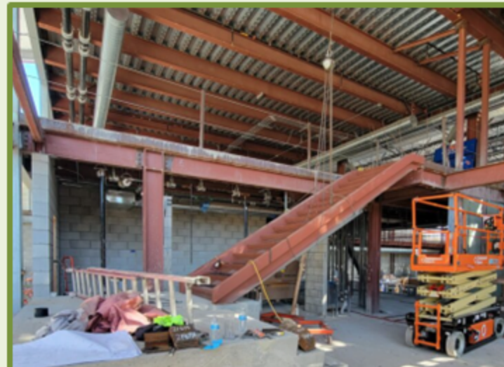
6 - Pool Lobby Stairs
