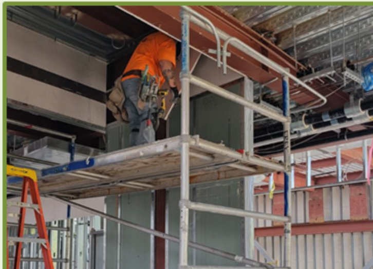
4 - Elevator Drywall Installation
