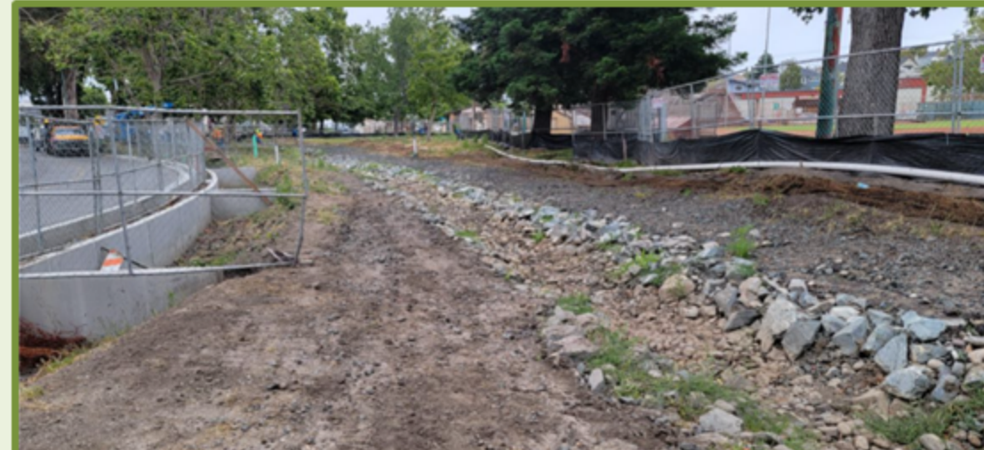
Irrigation Prep Work and Bioswale Clean Up
