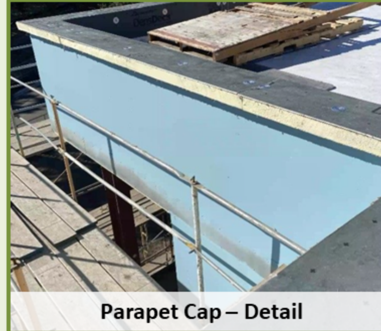
2 – Roof Insulation Board (1/2" To 2" Thick) Installation
