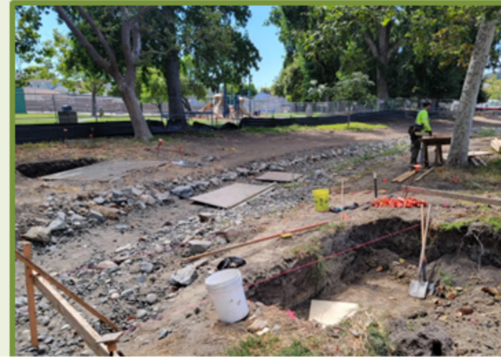
Pedestrian Bridge Abutment Formwork
