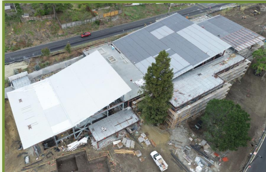
ROOFING WORK & INSULATION
