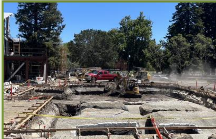
OUTDOOR POOL PLUMBING AND SHELL
