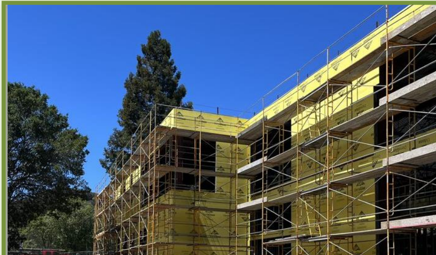
COMPLETE EXTERIOR WALL SHEATHING
