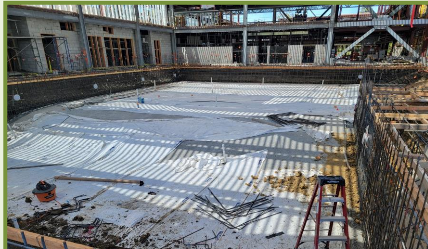
INDOOR POOL SHELL CURING
