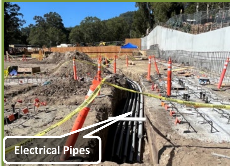
UNDERGROUND RELATED WORK (PLUMBING AND ELECTRICAL)
