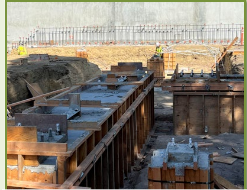
FOUNDATION STEM WALLS / ANCHOR BOLTS
