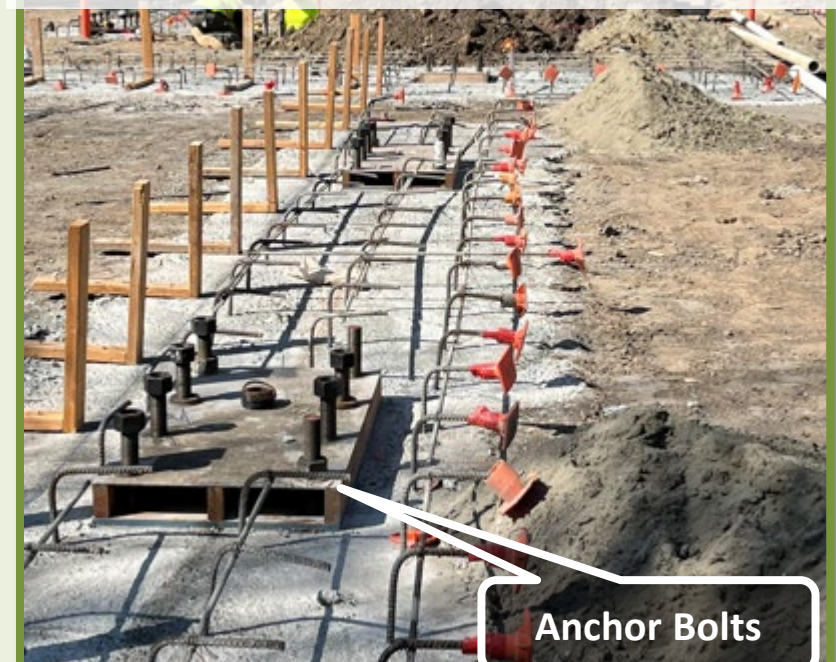
FOUNDATION STEM WALLS / ANCHOR BOLTS
