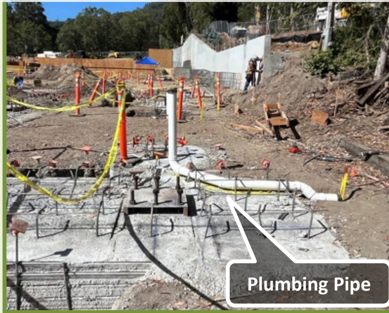
UNDERGROUND RELATED WORK (PLUMBING AND ELECTRICAL)
