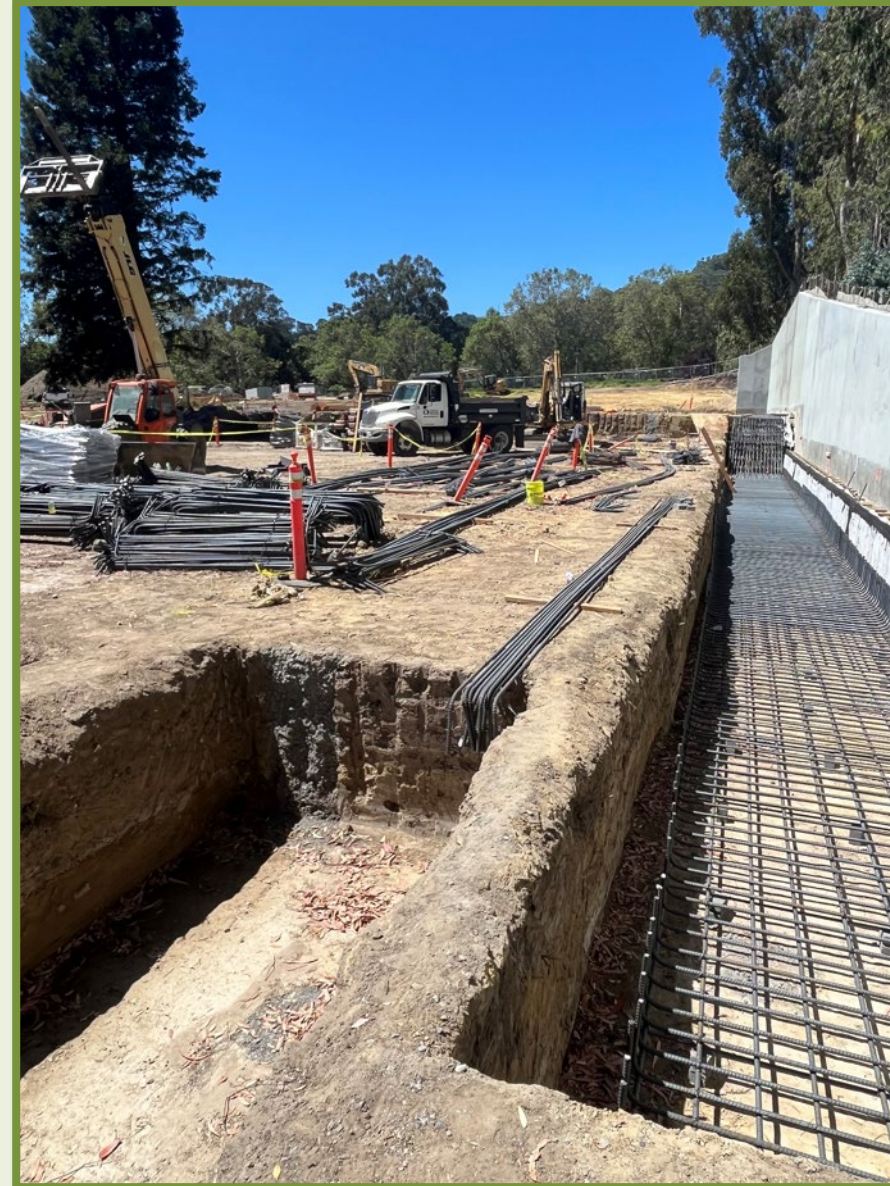
BUILDING FOUNDATION REINFORCING BARS
