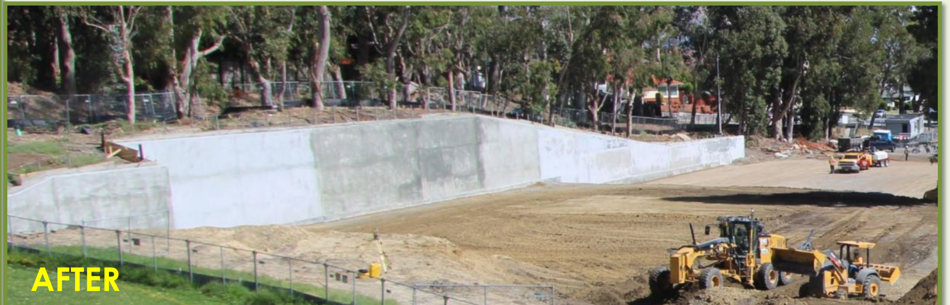
COMPLETED RETAINING WALL SURFACE, GEOPIER and BUILDING PAD
