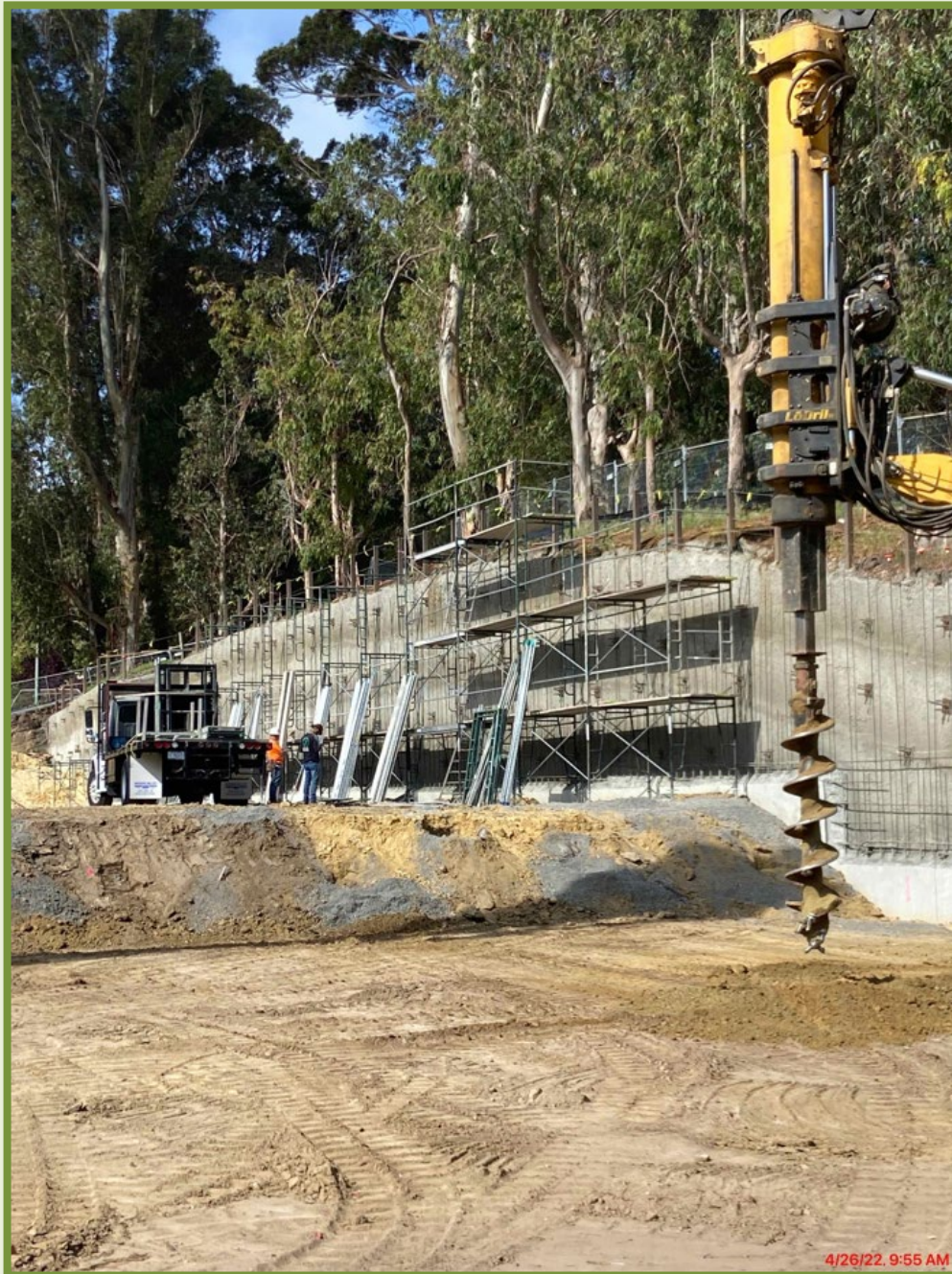
RETAINING WALL SURFACE AND GEOPIER
