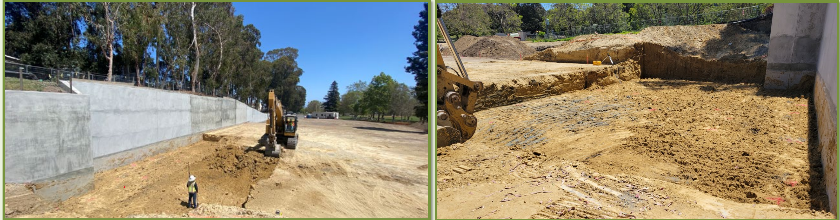
FOUNDATION WORK AT PUMP ROOM
