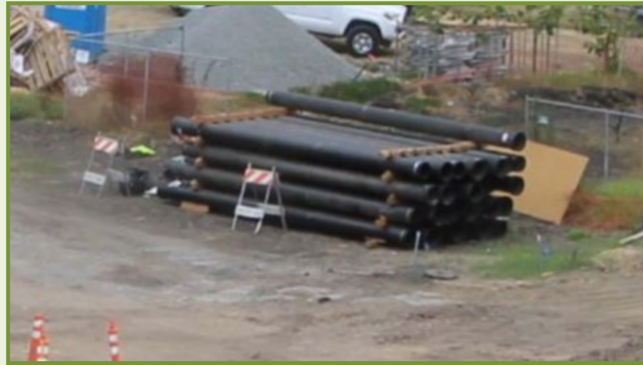
DUCTILE IRON PIPE DELIVERY
