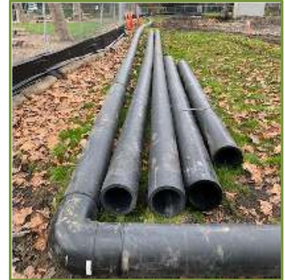
TEMPORARY WATER LINE BYPASS
