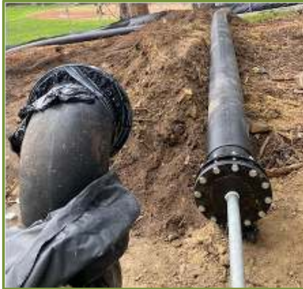
TEMPORARY WATER LINE BYPASS
