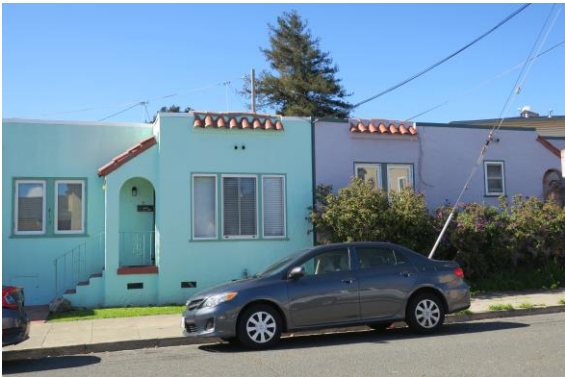
Figure 14: 415 and 413 San Anselmo Avenue North.
